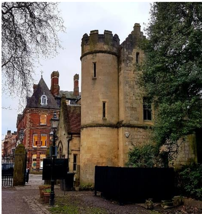
New bin screen next to YPS Lodge Photo: Steve Williams
